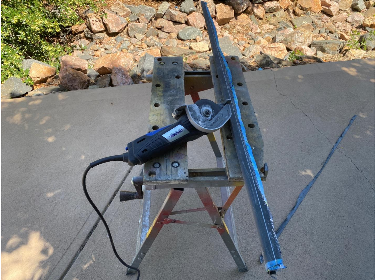
Above: Rough Cutting a frame piece
