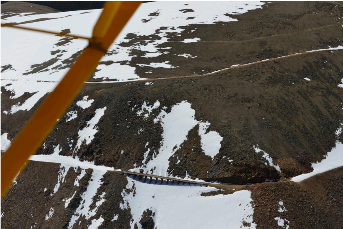
ABANDONED RAILROAD TRESTLES OVER ROLLINS PASS
